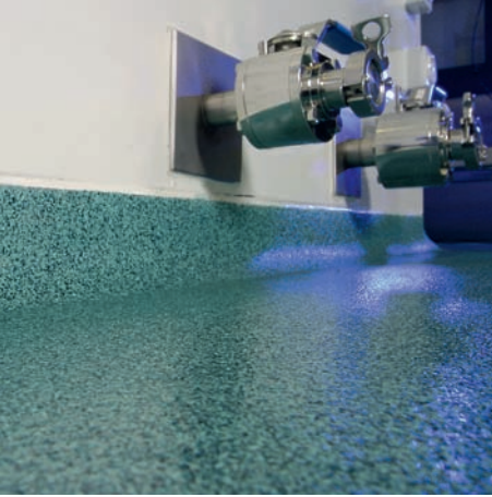
EPOXY SELF LEVELING WITH FLOOR FLAKES
