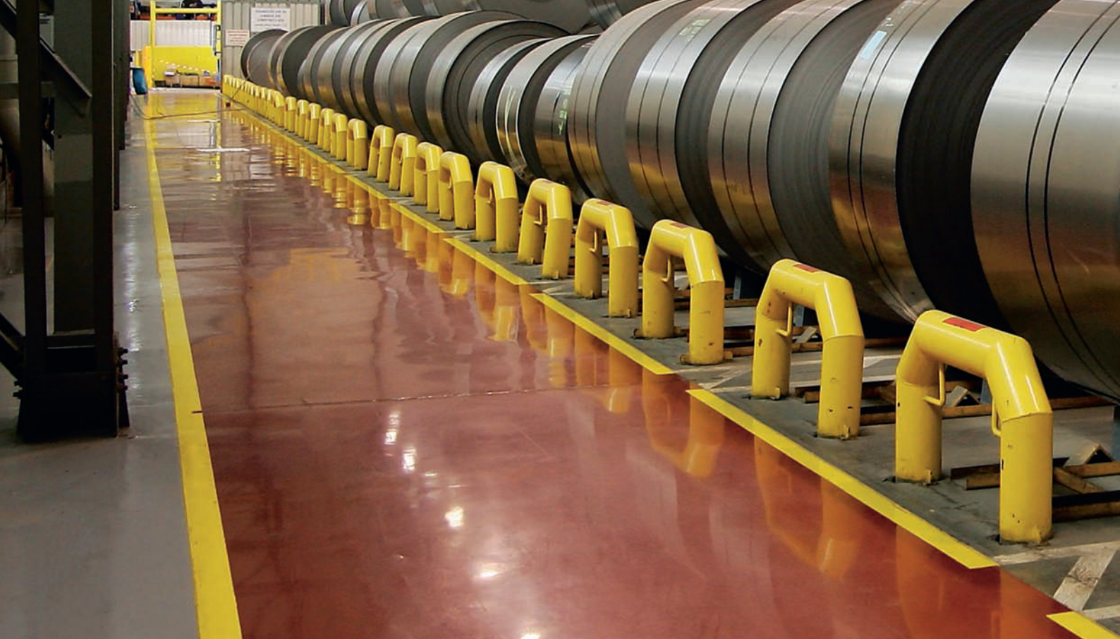
v EPOXY SELF LEVELING
